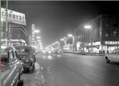
East Lake Street and Chicago Avenue, 1956
