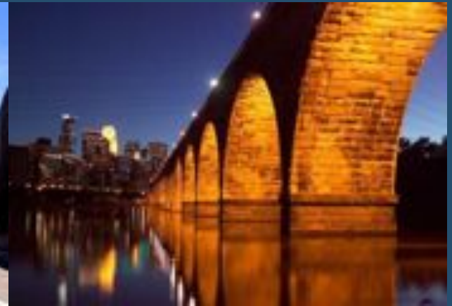
Stone Arch Bridge Restoration - Minneapolis
