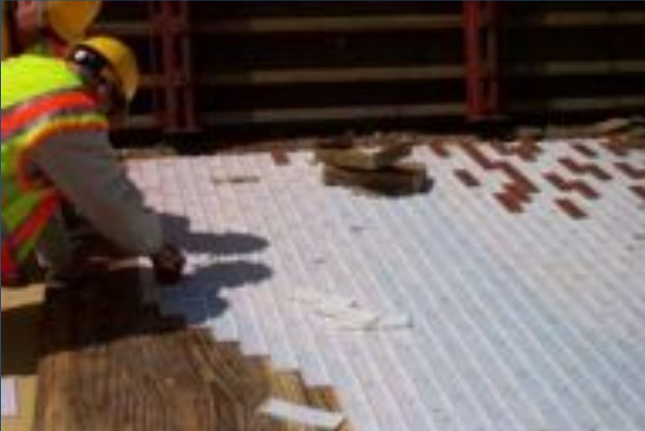
Thin Brick Installation
