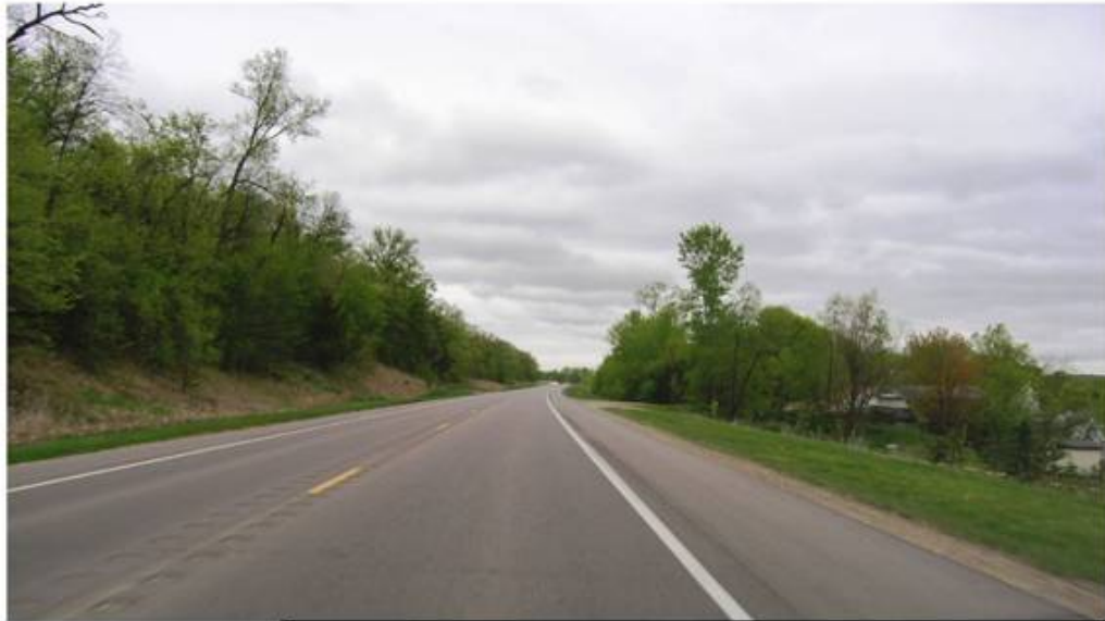
Existing US 14 - Next to Bluff (left) and Minnesota River Valley (right)
