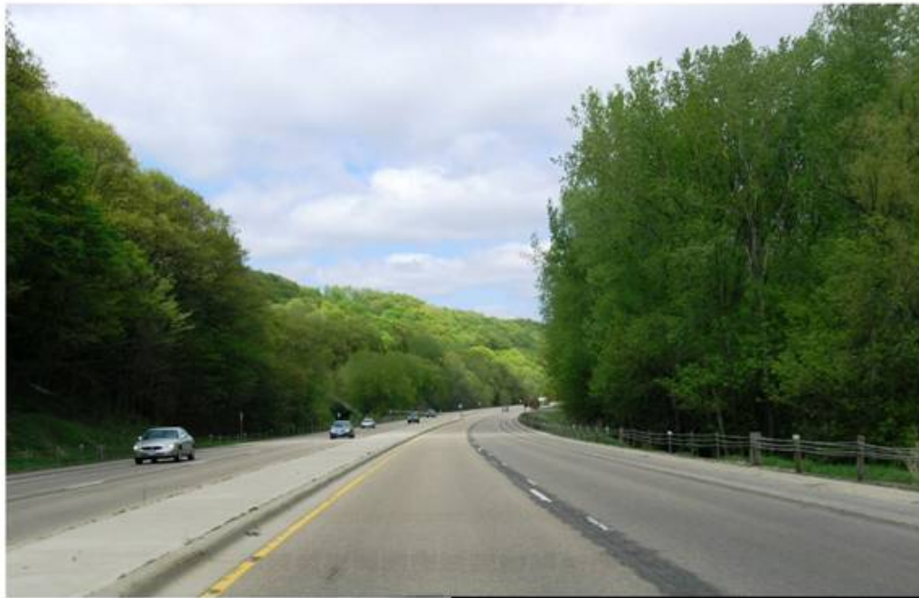
Existing US 169 South of St. Peter – Example of a 4-Lane Constrained Highway Design
