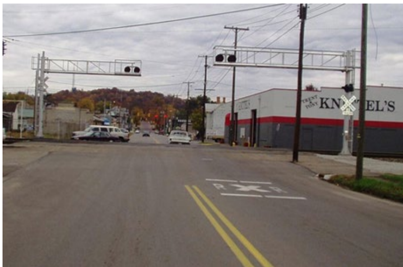
Figure 2. Typical Cantilever Flashing-Light Signals
