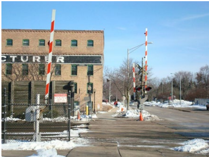
Figure 4. Standard Railroad Gates with Pedestrian Gates
