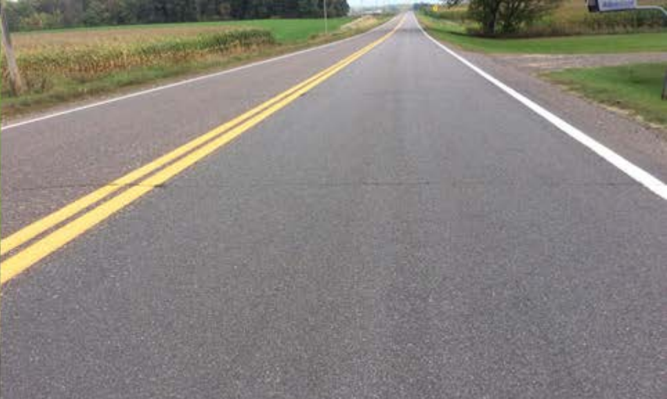
CSAH 8 eastbound Cell 11 Micro Surfacing Type II over Crack Seal / Transverse Mastic
