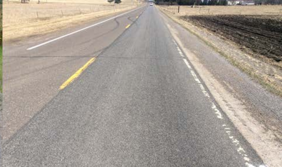
CSAH 8 eastbound Cell 6 Triple Chip Seal; FA 2 over FA 2.5 over CA-50/70
