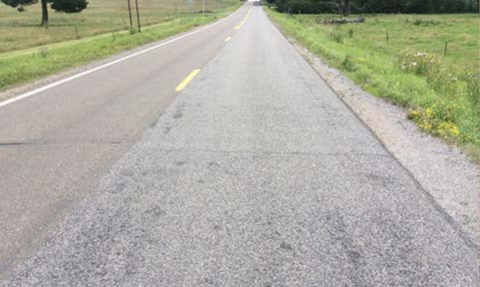
CSAH 8 eastbound Cell 7 Fiber Mat Chip Seal FA 2.5
