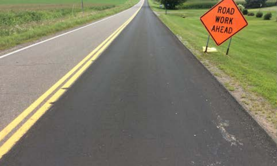
CSAH 8 eastbound Cell 11 Micro Surfacing Type II over Crack Seal / Transverse Mastic
