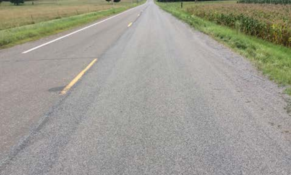
CSAH 8 eastbound Cell 6 Triple Chip Seal; FA 2 over FA 2.5 over CA-50/70
