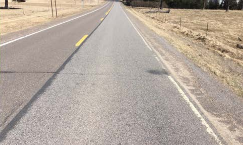
CSAH 8 eastbound Cell 7 Fiber Mat Chip Seal FA 2.5
