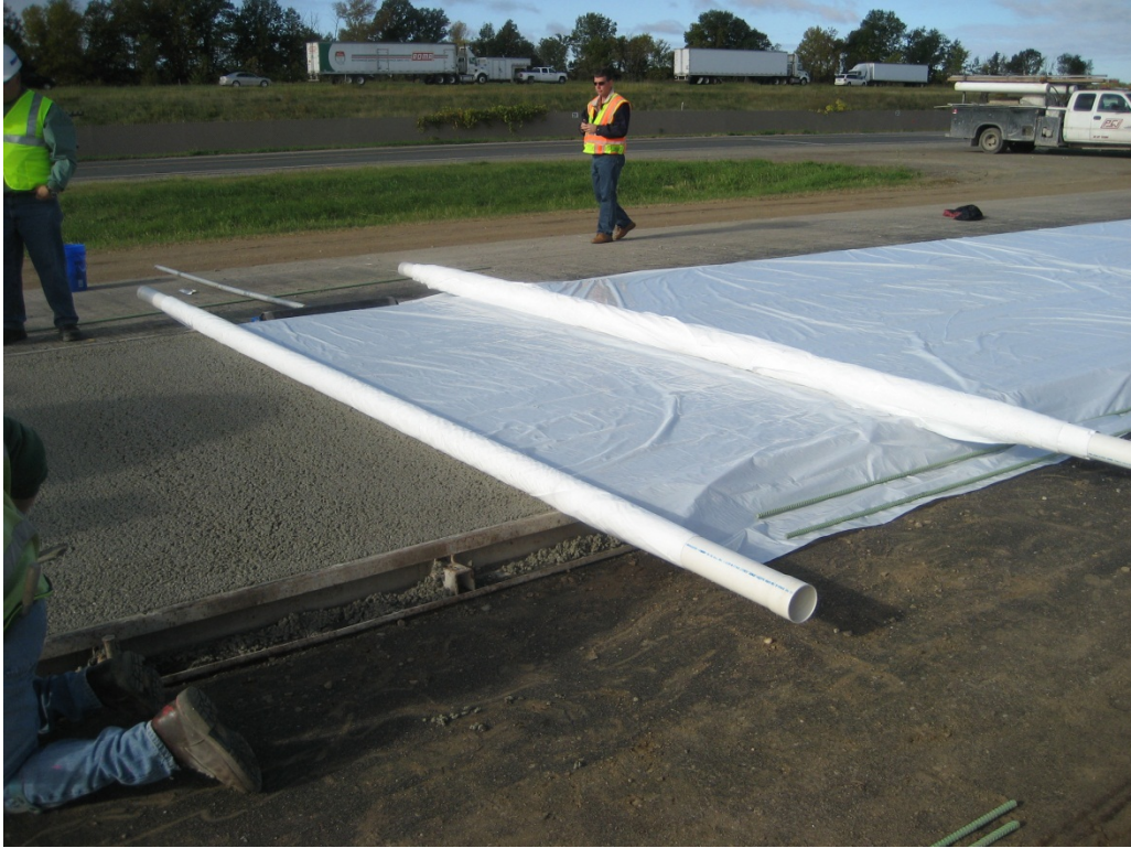
Figure 60. Completed surface of pervious overlay and covering with two layers of plastic
