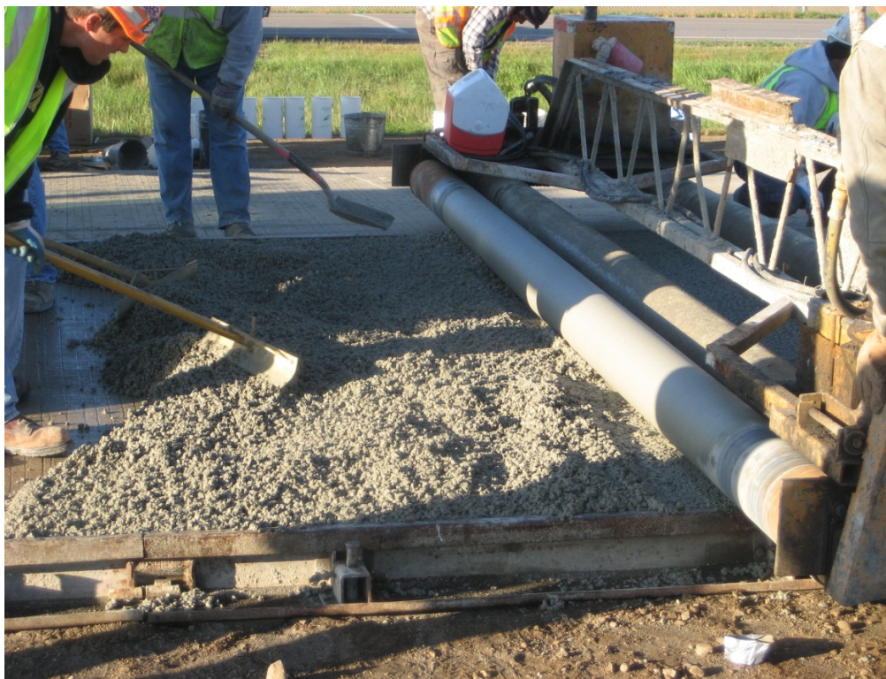
Figure 59. Placement of pervious concrete overlay using roller-screed
