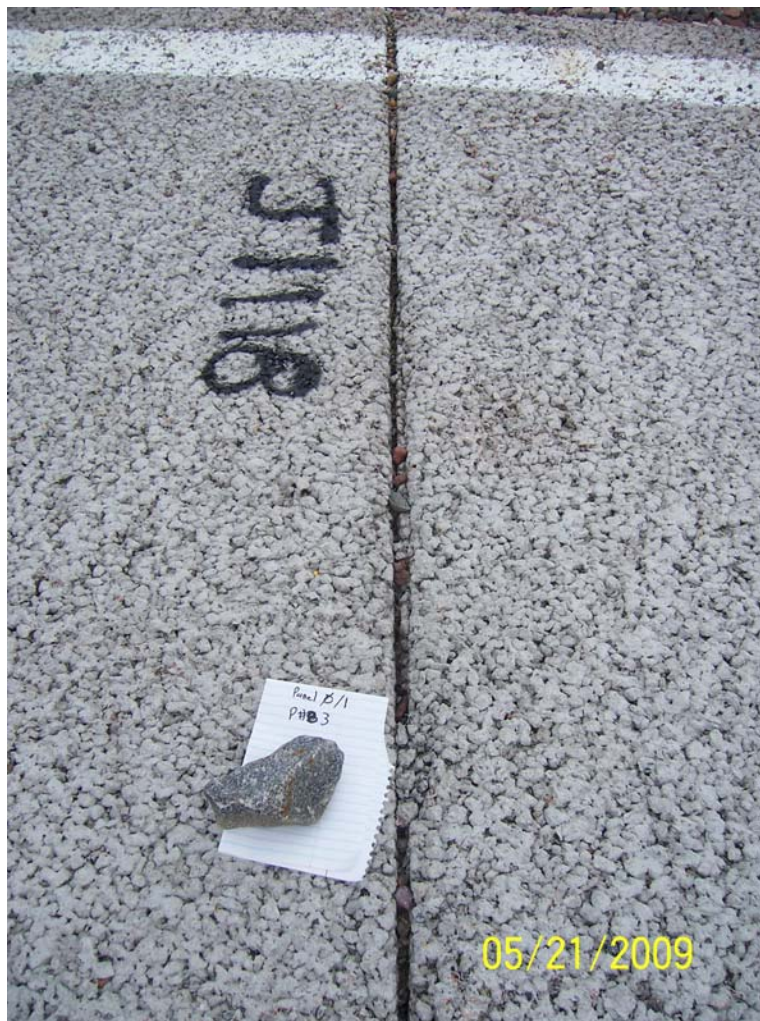
Figure 70. Example of double-jointing
