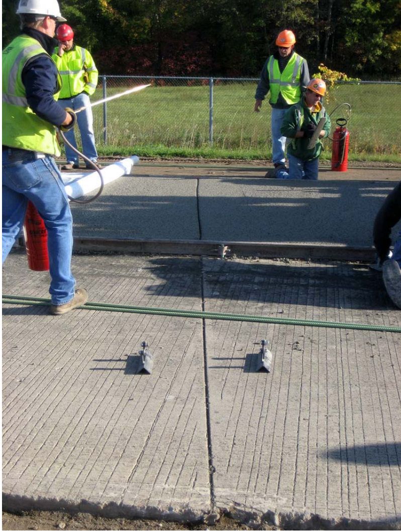
Figure 72. Jointing on fresh pavement
