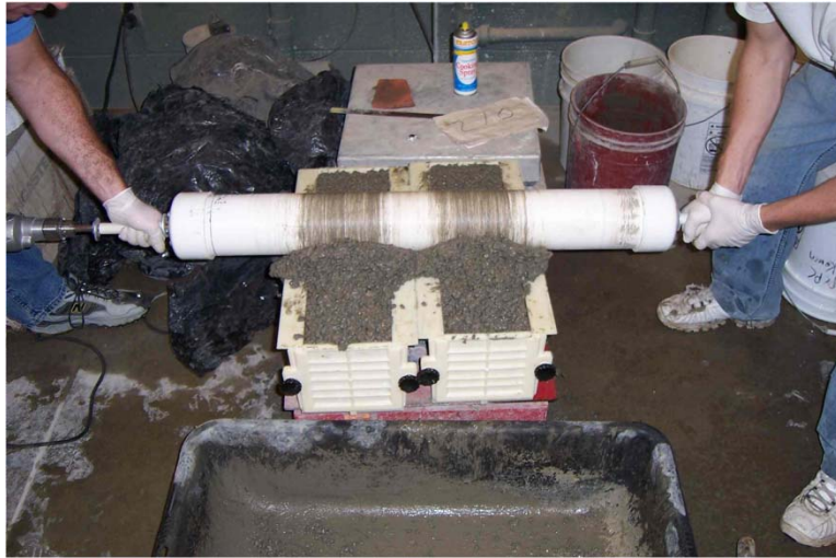
Figure 35. Finishing using a roller screed
