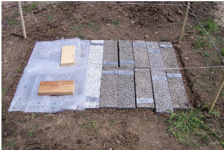
Figure 38. Initial beam curing
