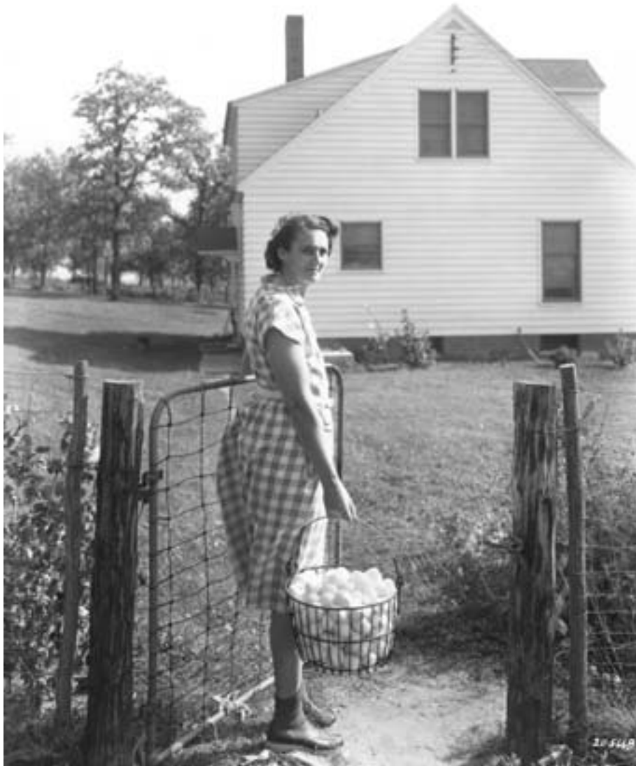
This woven wire fence had wooden posts and a steel gate. Location unknown, 1952. (MHS photo by Norton and Peel)
