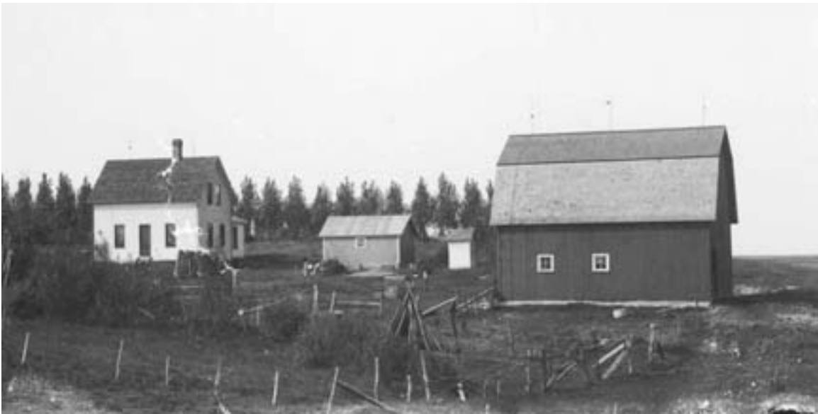
This moderately-sized general purpose barn had vertical siding and three lightning rods on the roof. Location unknown, circa 1900. (MHS photo by John T. Austinson)
