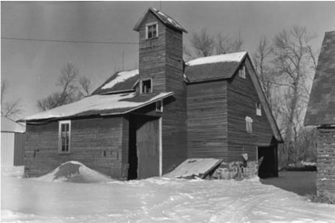
Built circa 1885, this farm elevator had woodframe construction, clapboard siding, a scale for weighing, and elevating equipment that filled at least seven overhead bins. The elevator was also used for machinery storage. Twente Farm, Brown County, 1979. (MHS photo by Gimmetstad)
