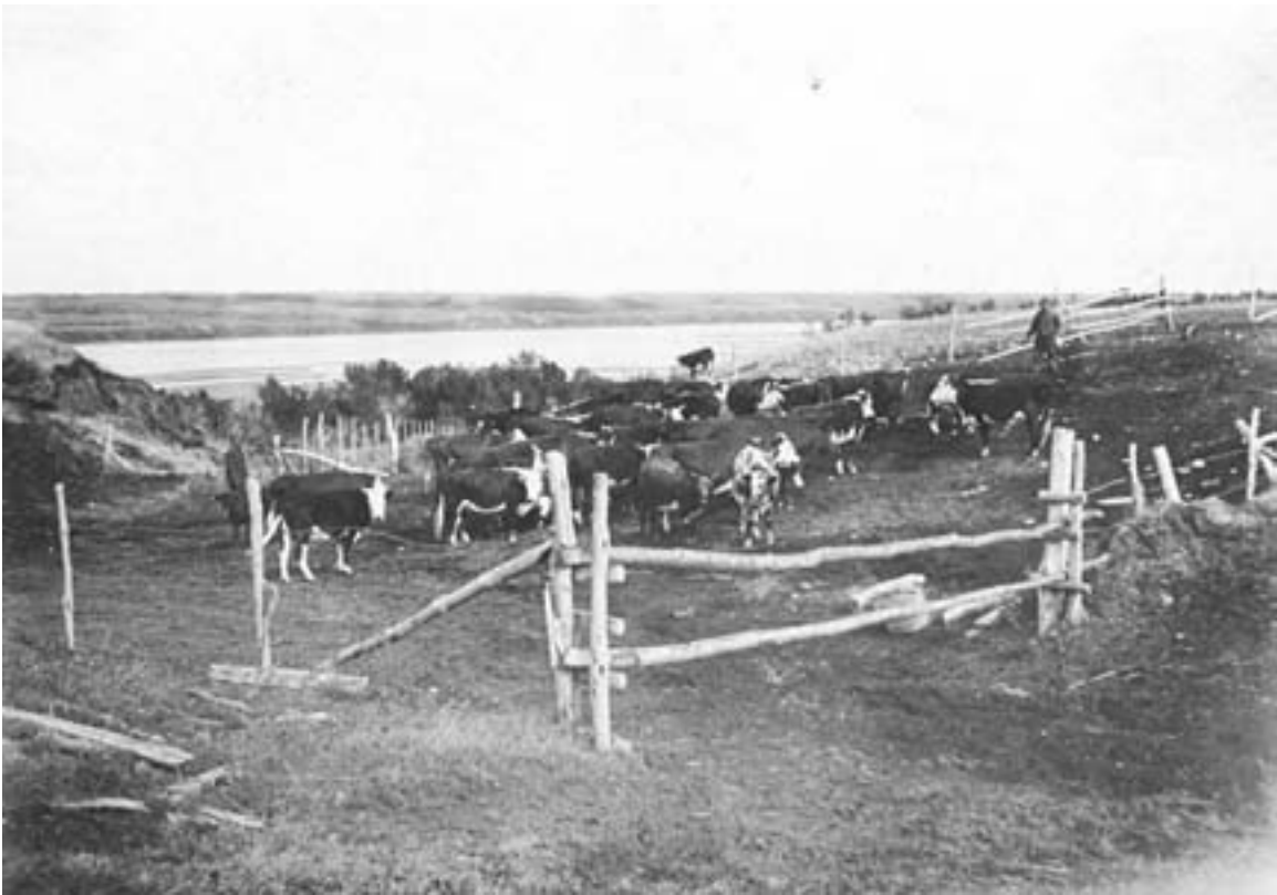
A barbed wire fence with a braced corner post and a simple gate consisting of two removable log rails. Farmers tried to plan their fields so they didn't have to open and close too many gates as they moved machines or livestock from field to field. Location unknown, circa 1910. (MHS photo)
