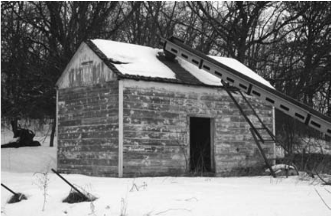
Portable elevators or conveyors became available around 1904 and were widely used throughout Minnesota. Granaries were filled through hatches located in the roof or upper walls. This granary probably has two bins. Fillmore County, 2001. (Gemini Research photo)
