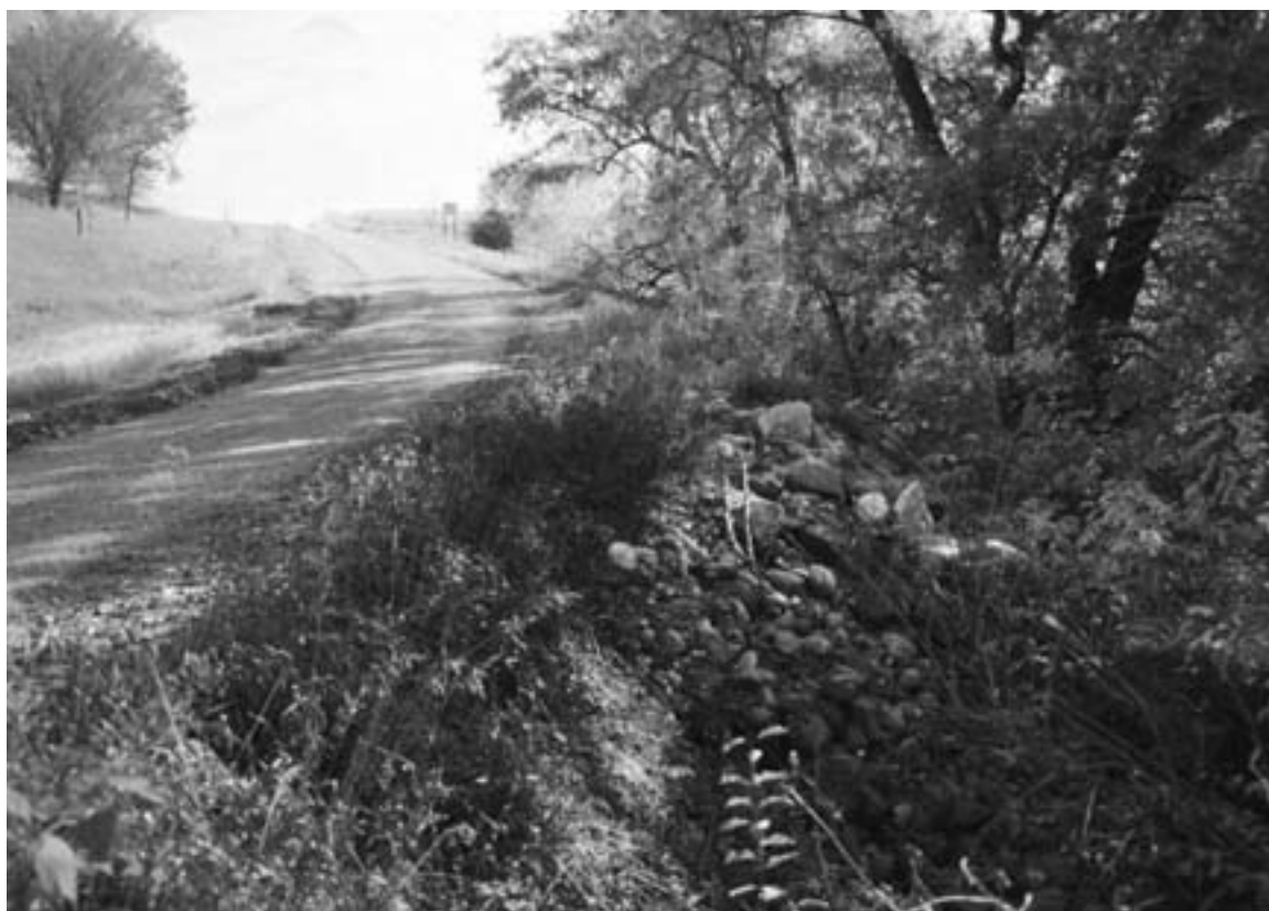
It was common to pile field rocks at the edges of roads or streams to serve as ripraping. Retzlaff Farm, Framnas Township, Stevens County, 2004. (Gemini Research photo)
